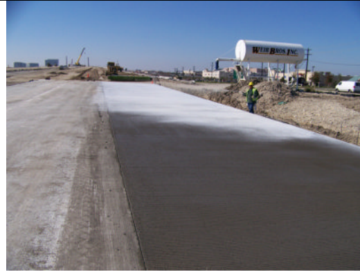
Figure 10 – Curing Compound
