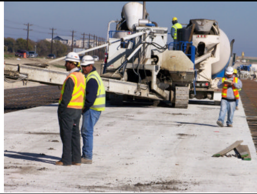
Figure 4 - Paving Train
