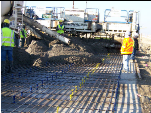
Figure 3 – Paving Train
