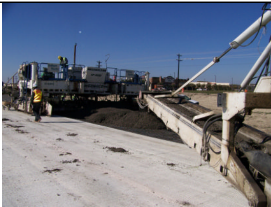
Figure 5 - Paving Train
